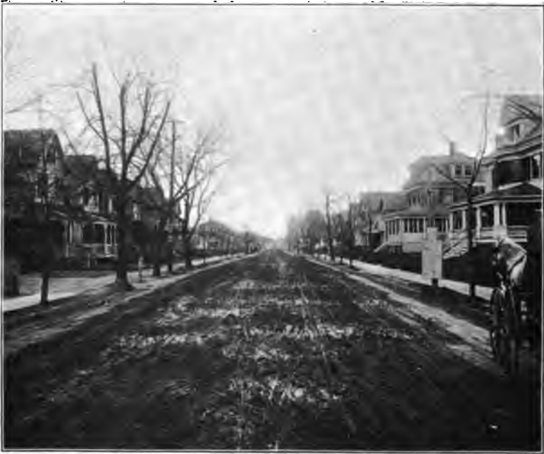
Corliss Avenue, Monmouth Co., before improvement.
